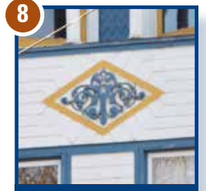
8 619 - 621 West Water Street
