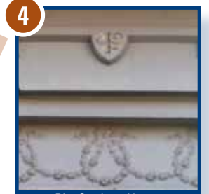
4 Ritz Carriage House 359 W. Clinton Street
